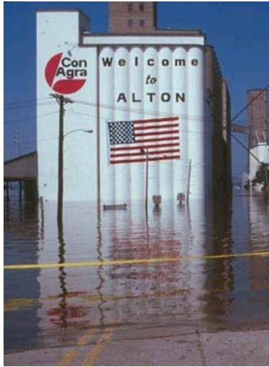
ConAgra plant during flood of 1993 - it sits across the street from the new flood memorial.
